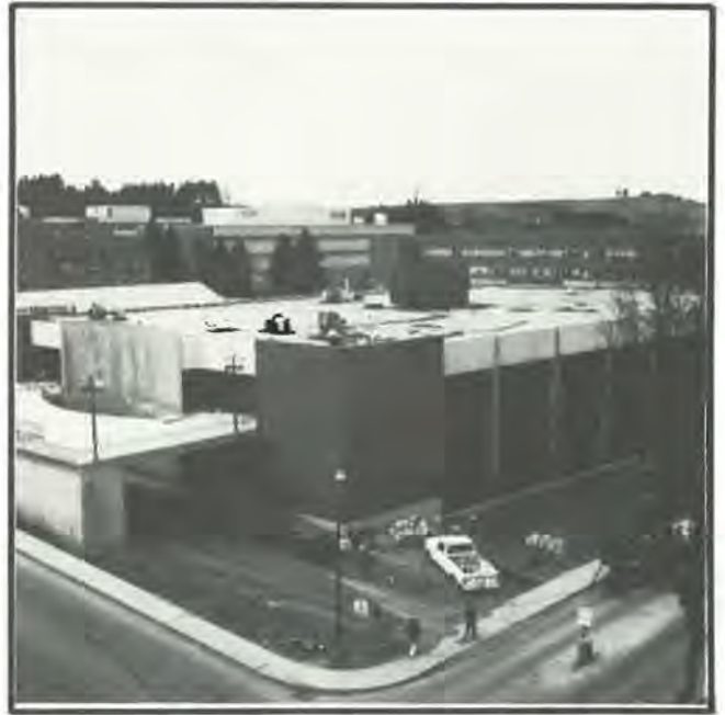
FWR Building under construction, 1971.
