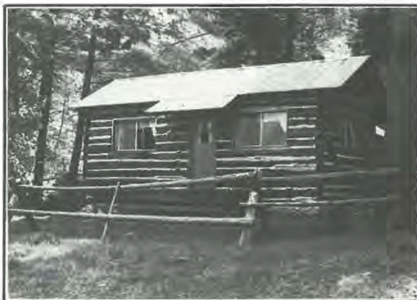
Still in use is the cabin of “Cougar Dave” Lewis, the original occupant of Taylor Ranch. The cabin now houses scientists conducting research in the Frank Church-River of No Return Wilderness.
