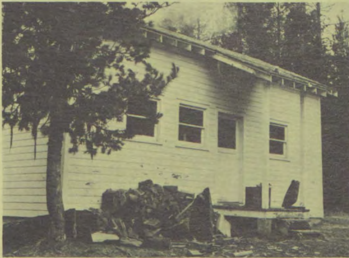
Rustic cabin provides temporary home for loggers and researchers working on the College Forest.
