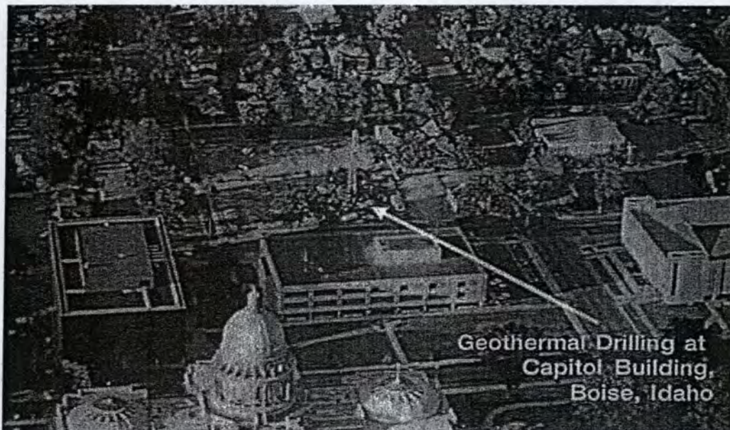
Figure 2.19 The Idaho Capitol Building Complex is Heated from Geothermal
