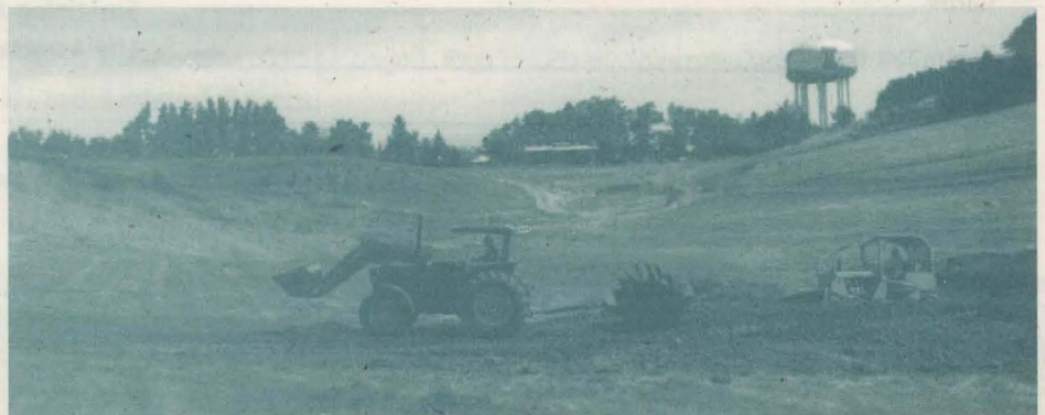
Pond construction, summer 1986. Equipment furnished by Eugene Thompson.
