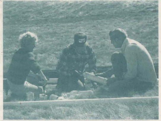
Laying pipe, October 1984. L-R—Jayne Cronk, R.J. Naskali, and Bob Bullock (GTE).
