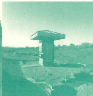
A Keystone and brick overlook deck nears completion.
