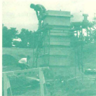
A&R Construction personnel prepare the forms (8/14/97) and pour the cement (8/18/97) for the kiosk core.
