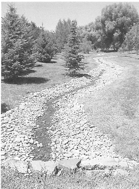
New rock was added to the beds of the stream that runs through the Arboretum. The rock was added to help with erosion. Charles Zillinger photo August 15, 2003
