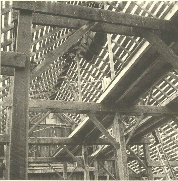
The superstructure of the hayloft after the worn cedar shakes were removed prior to re-sheathing the roof deck as viewed toward the gable's roof vent opening. Note the scaffolding and ladders with contractors raising the gable peak to its original height. Photo February 3, 1998 by R.J. Naskali.
