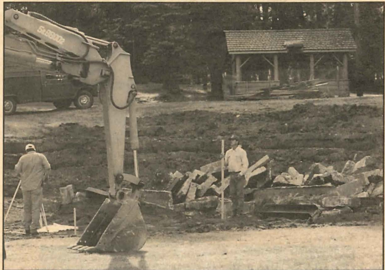
Demolition of the amphitheater in the Charles Houston Shattuck Arboretum, September 6, 2001.
