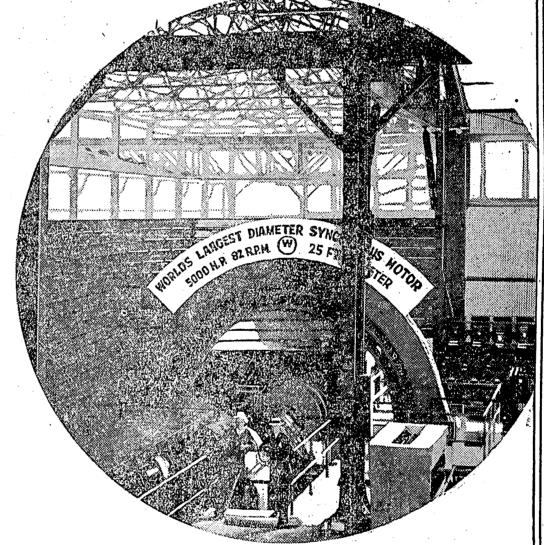
This 5,000 h. p. motor in the Columbia Steel Company's plant, with its frame of arc-welded steel, is physically the largest synchronous motor ever built.
