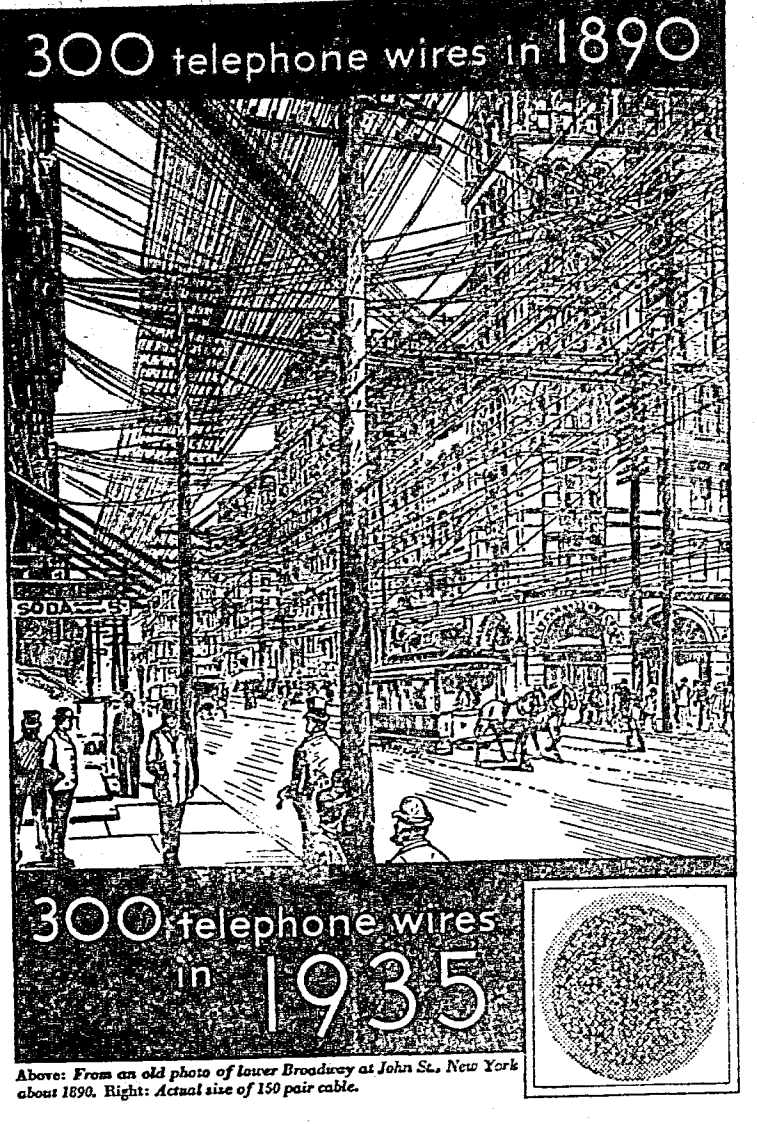
300 telephone wires in 1890 300 telephone wires in 1935 Above: From an old photo of lower Broadway at John St., New York about 1890. Right: Actual size of 150 pair cable.
