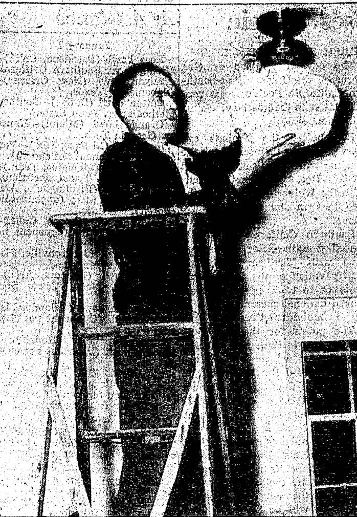
Shown attaching a ceiling fixture to a light bulb in one of the university's temporary classroom buildings is Henrik Juve, university electrician. Student and faculty requests alike prompted the change to better, diffused lighting in the buildings, which was carried out during the weekend.
