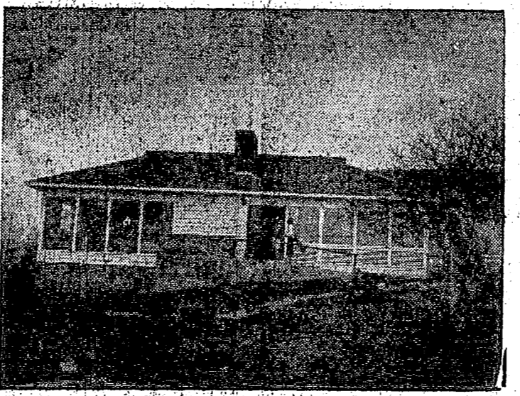
The newly-completed golf club house has been a mecca for golfers and loungers alike. The new building includes showers, cafe, lounge with full length windows and a pro shop. The grand opening of the ASUI project was held April 2.
