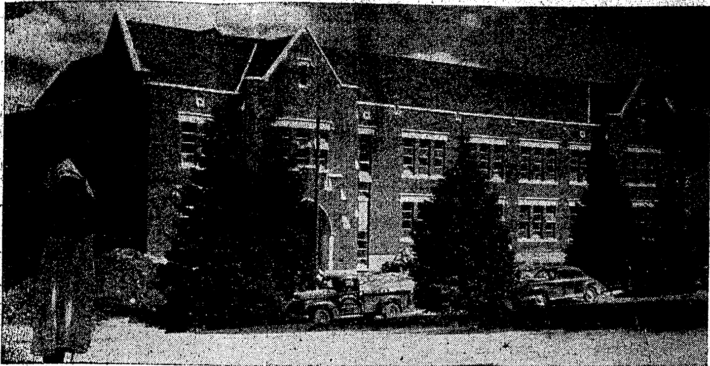
Idaho's new Music building, when completed soon will give University musicians a real place to call "home" instead of wandering among the five wooden cottages previously used as music headquarters. Here Nancy Shelton surveys while finishing touches are in the offing.
