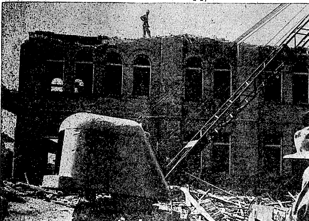
Removed during the summer, the old Engineering building was one of the last old campus landmarks. Prior to its destruction, the building was the oldest building on the campus. It was torn down to make way for a new Home Economics building.
