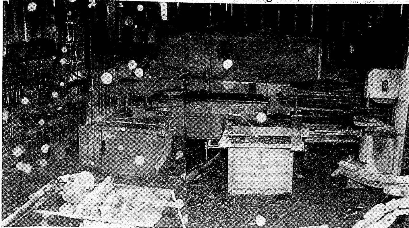
An early morning fire yesterday razed the interior of the northwest wing of the Industrial Arts building, causing an estimated $20,000 damage. The interior of the wing (shown above) was gutted by the fire first reported at 2:20 a.m. yesterday morning. The
