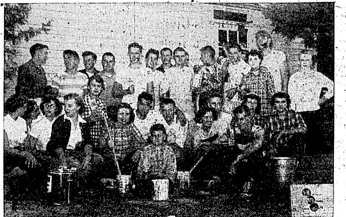
Giving a helping hand in the renovation of the Idaho club are these students from the university, as well as a few maidens from across the state line. The reason for the "paint party" was to give the Idaho club a new face inside and out. Entertainment followed the day of hard work.
