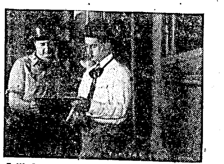
E. W. Griffin, B.S. in M.E., Duke; M.S. in Ind. Mgt., Georgia Tech '52 (right), instructs operator in handling of super-light horizontal vacuum filter used in separating adiponitrile from sodium chloride.
