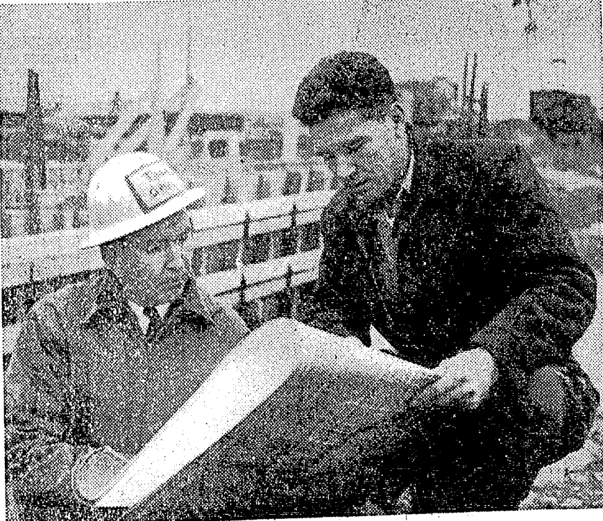
Cliff Downer (right), A.B. in Mathematics, '49, M.S. in Civil Engineering, '50, Harvard, on the site of a building construction project.
