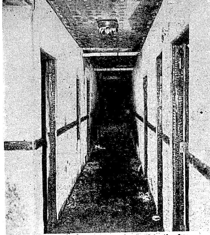
resulting in $100,000 damage. Extreme left photo is of the west wing of Gault Hall after the fire. The large windows on the second floor are at the front of the lounge. The windows on the third and fourth floors are in students rooms. Center photo is of the fourth floor hallway where two of the students bodies were found. One body
