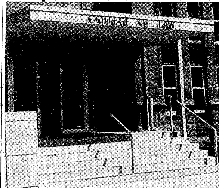
This is the entrance to the new facilities for the College of Law located in the south wing of the Administration Building. Renovation of the interior of the building is still in progress.
