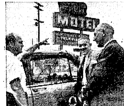
"1:30 p.m. After lunch, I look in on a PBX and room-phone installation at an out-of-town motel. The installation supervisor, foreman and I discuss plans for running cable, in from the highway."
