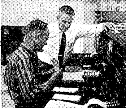
"9:30 a.m. The State Police at Andover have reported trouble with a mobile radio telephone. I discuss it with the test deskman. Naturally, we send a repairman out pronto to take care of it."
