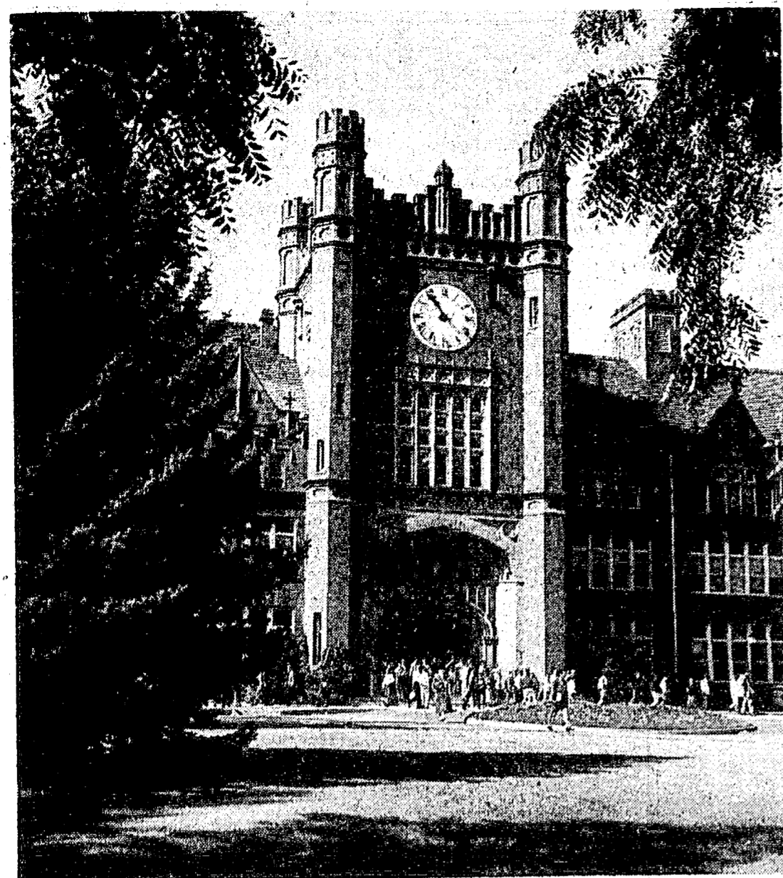
THE CLOCK STOPPED — The clock in the Administration Building tower, landmark at Idaho since 1913, is reliable most of the time, but it stopped briefly and underwent minor repairs during Christmas vacation. The clock has a long, interesting background of stops and starts.
