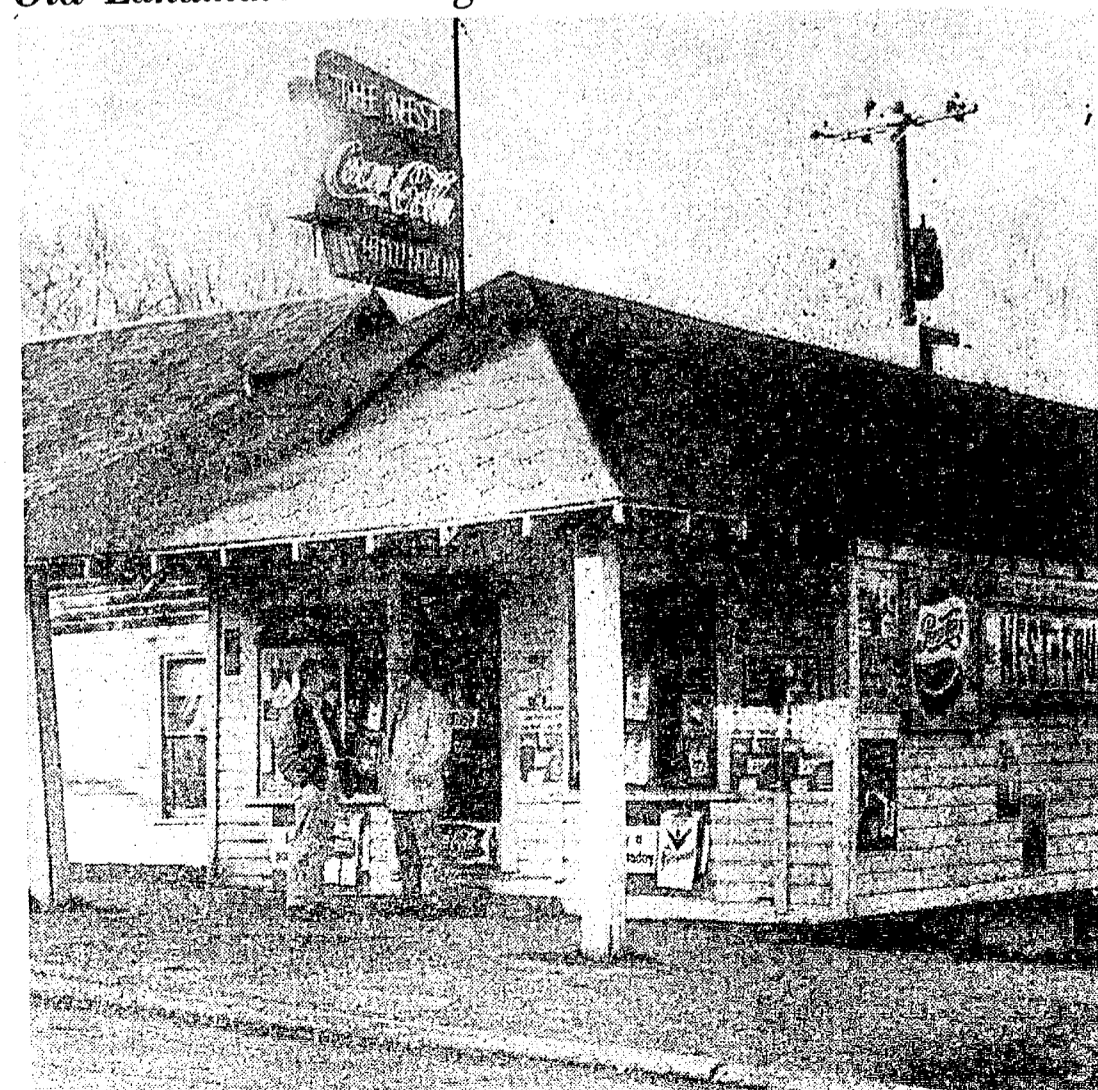
PROGRESS calls for the tearing down of the Nest. The building will be torn down so that a new, safer approach to campus can be made. No immediate plans for destroying the Nest have been made yet, however.
