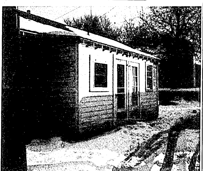
ALLEY FRONTAGE NOT ALLOWED? — Moscow City Zoning Ordinance: "A dwelling shall front a public street. Alley frontage will not be allowed." Section 4-4-16.
