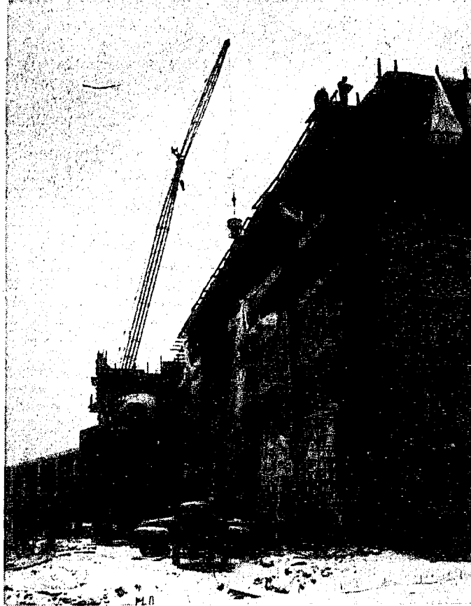
NEITHER RAIN NOR SNOW — Nothing seems to halt the pace of the construction on the Wallace Dormitory addition. Taking on a final shape, the building is scheduled for completion before school starts next fall.
