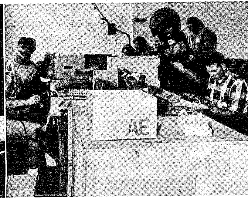
Even packing crates serve as work benches as installation crews tackle re-construction tasks.
