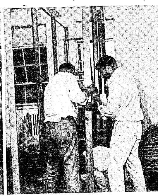
Meanwhile, crews in the central office were busy installing racks to hold the new switching equipment.
