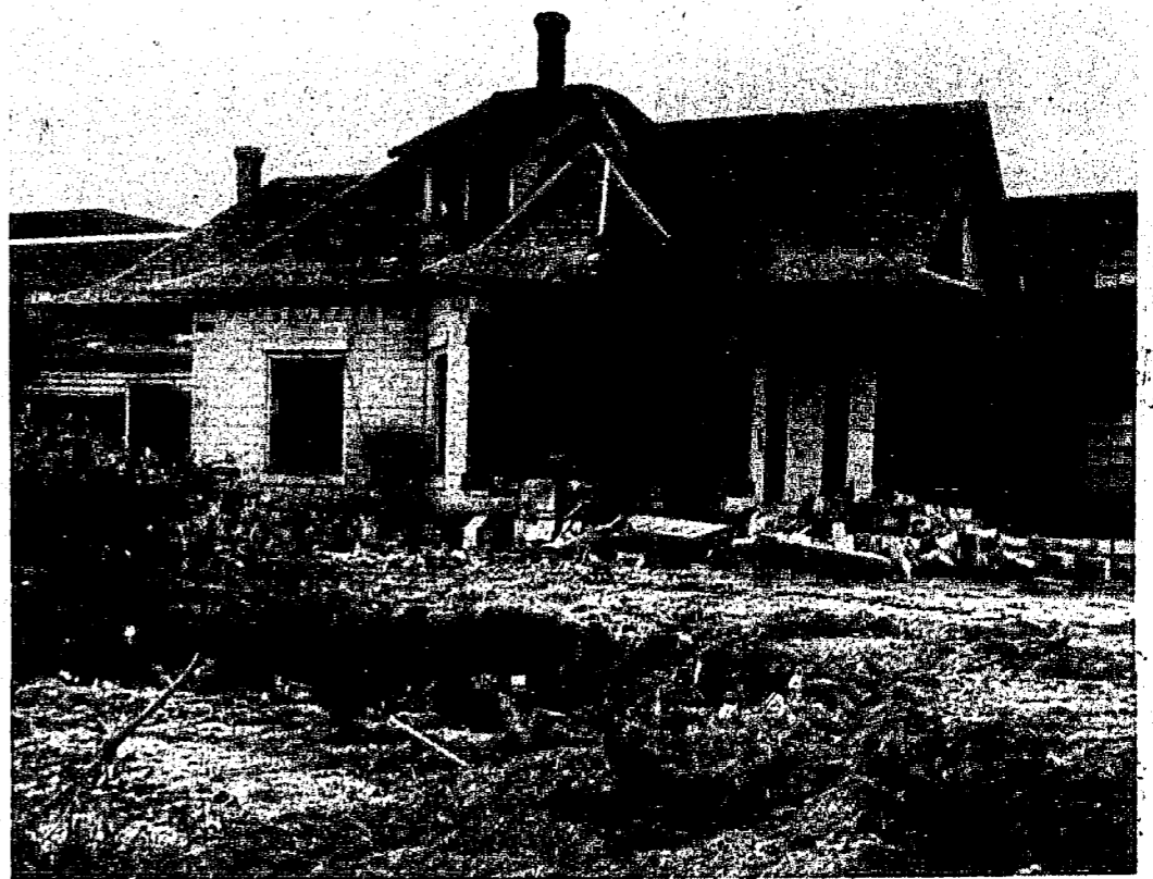
FIREWOOD —Tear down the old and make way for the new is the philosophy as wreckers tear this building down in order to make room for the new addition to the Kirtley Laboratory. The Rally Committee has torn down one of the buildings and will burn the remainder tonight at the rally.
