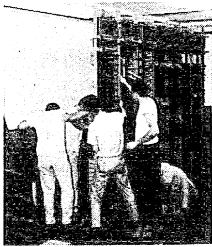
Another panel goes into place, ready for installers to start connecting thousands of wires. This crew has men from all parts of the Northwest.
