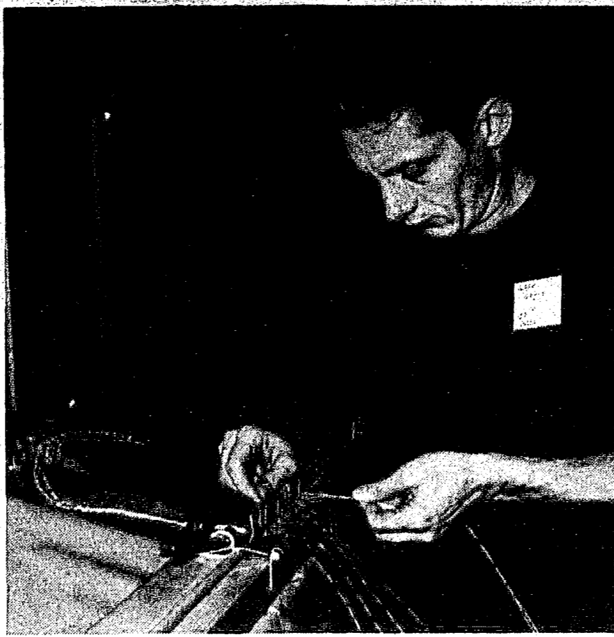
Gary Getty, from Gen Tel's Everett staff, codes the wiring to be installed in new switchboards.
