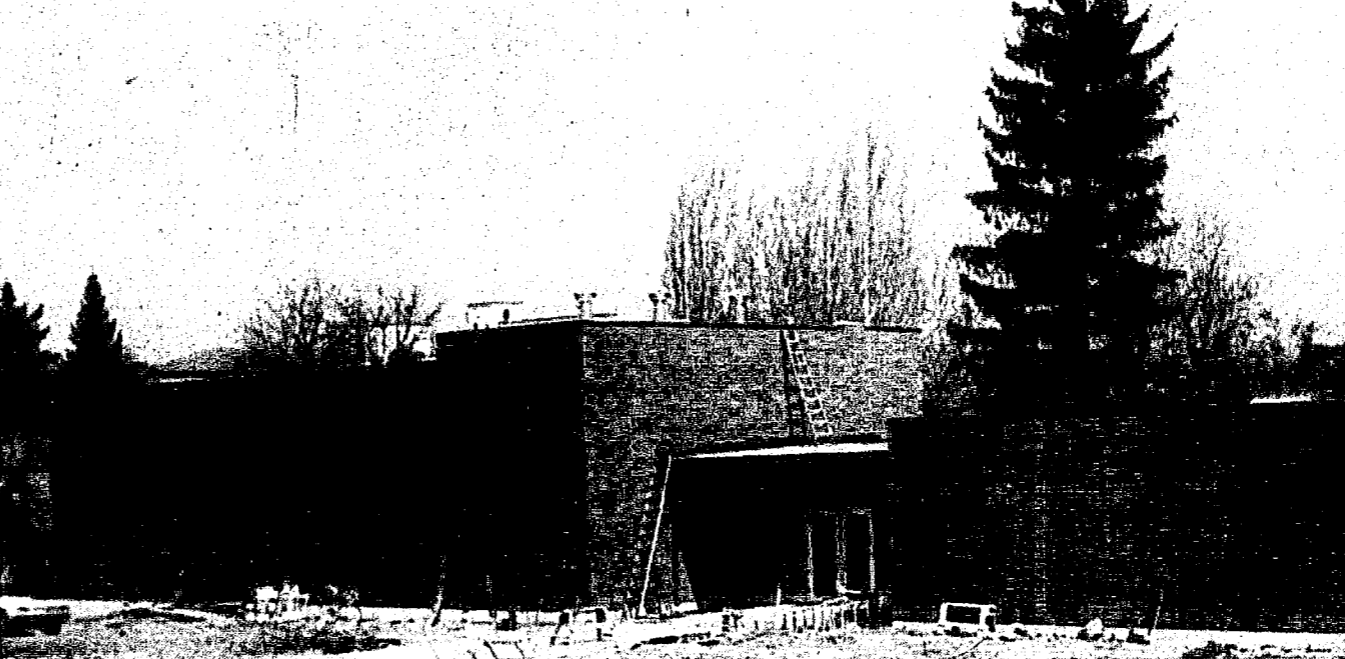
THE LDS INSTITUTE, which is near completion, was dedicated last Friday at a noon ceremony by Dr. Ernest Hartung, president of the University. The building, which cost $230,000, held its first service Sunday. (Bower photo)
