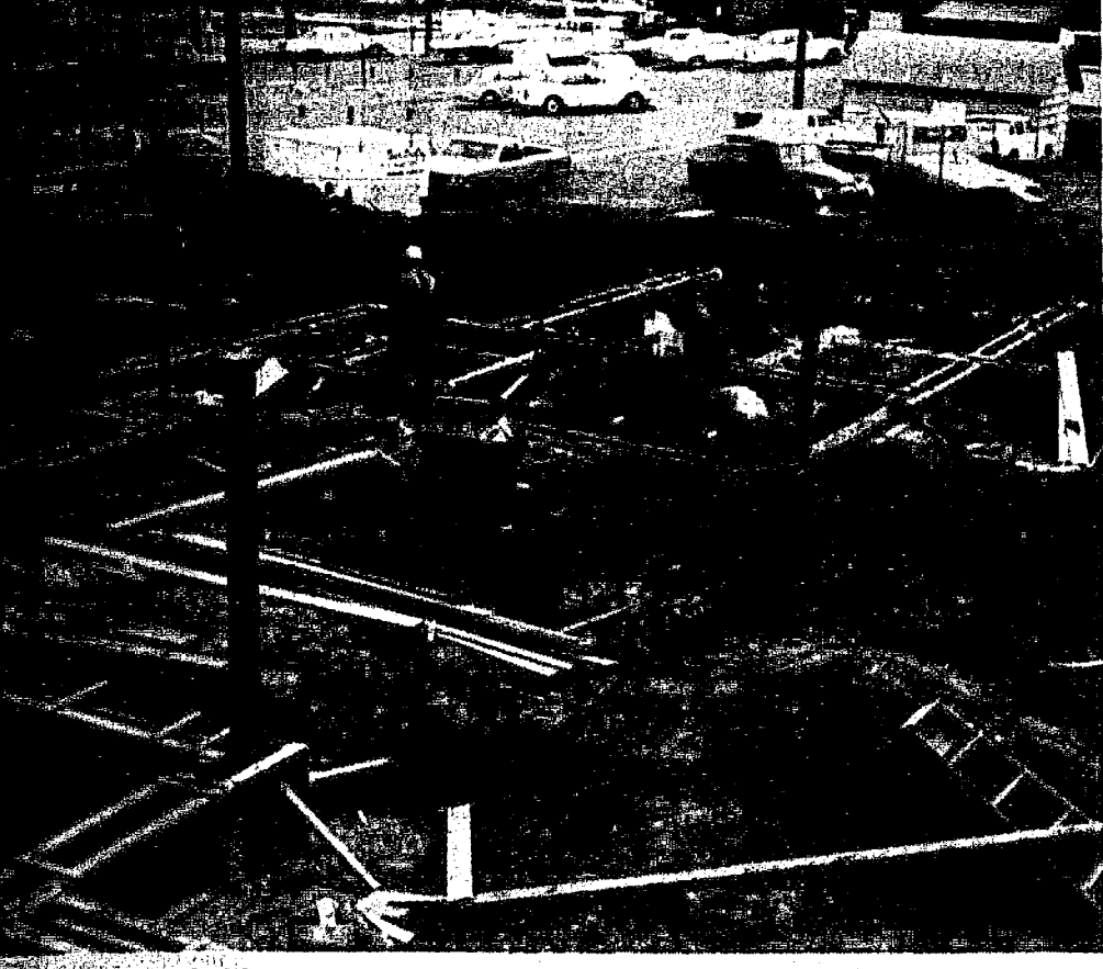
FOUNDATIONS OF THE PHI DELTA THETA House have finally begun to take shape after a strike at the University halted work for about two weeks last month. Completion date for the new house will be around the first of September. The Phi Deltas are presently living in Pine Hall.—(Bower Photo)
