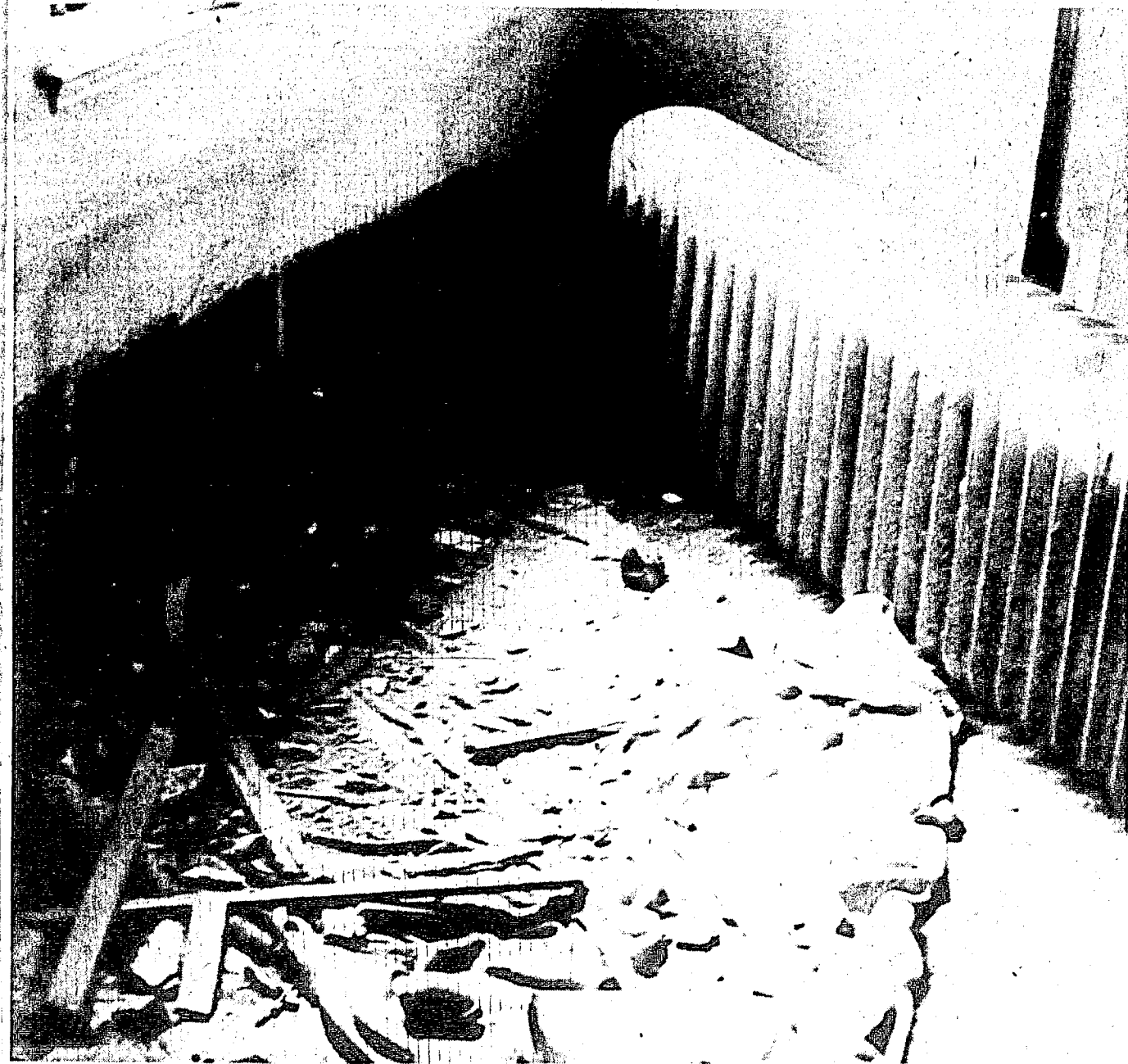
WATER DAMAGE—A little bit of plaster and a score of useless radiators are all the Lambda Chis have to show for the sub-zero cold that hit Moscow during the Christmas vacation. Several other fraternity houses, dormitories and class room buildings were damaged by water when the temperatures raised and the results of the minus 40 degree weather became known.
