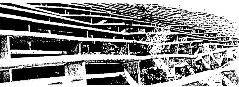
IDAHO'S BLEACHERS ARE FALLING DOWN, falling down — Bleachers in Neale Stadium have been condemned. A survey by engineers showed the 32-year-old facility to be unsafe for football action this fall. Idaho's home games will be played on the WSU field.
