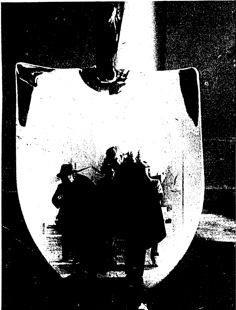
GOVERNOR DON SAMUELSON and President Ernest Hartung turn over the first shovelful of earth in the official groundbreaking ceremonies in January for the new Forestry Building. The area now appears as a large hole in the ground, with foundations going in rapidly.
