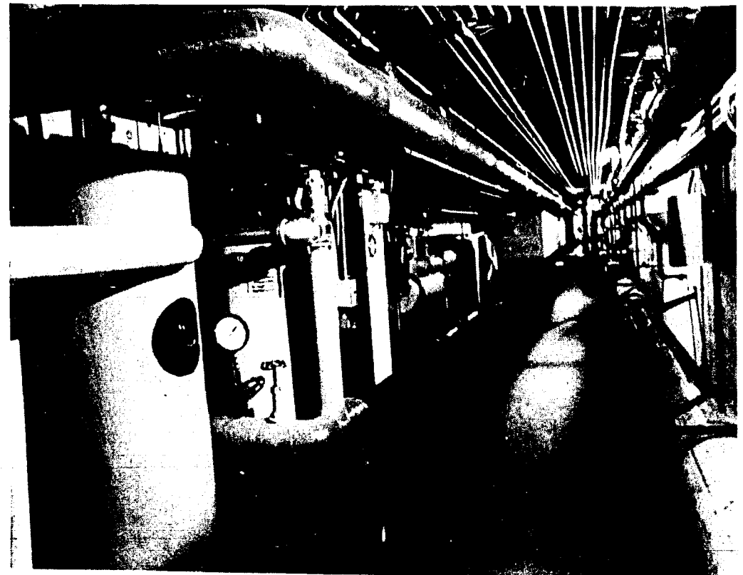
Color-coded pipes, and a new filter system are only part of the maze of pipes that keep the pools in operating order.
