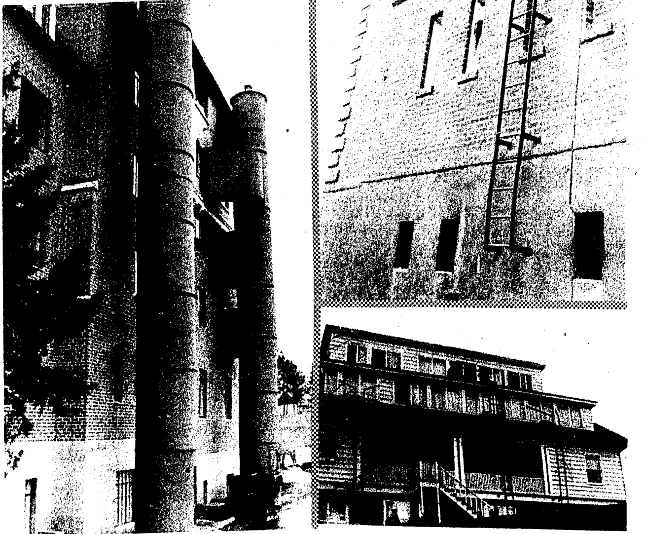
OF QUESTIONABLE WORTH — A locked fire-escape chute, a wooden frame building, a vine covered fire-escape and a fire escape that ends six feet from the ground all are of questionable fire safety. The fire escape
