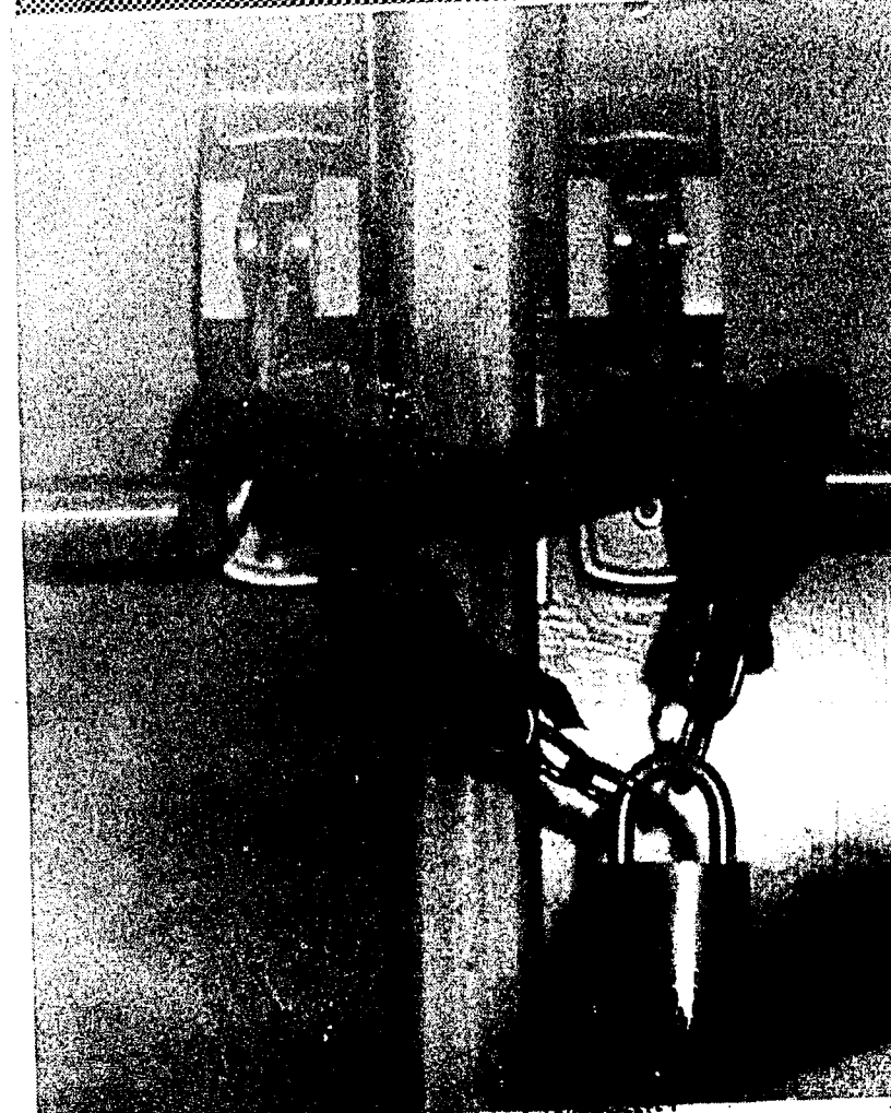
THESE DOORS are the only exit in the SUB basement which lead directly to the outside. All doors in the SUB are locked nightly—these doors, located just outside the Argonaut and ASUI senate offices, are padlocked just after closing. In the event of a fire, and the smoke which results, the 11 students who spend at least two evenings a week in the SUB basement would be trapped. When questioned about the reason these doors are padlocked (they have been altered anyway so that only an exit is possible) Student Union Building officials said, "We've had a great deal of trouble with thefts."
