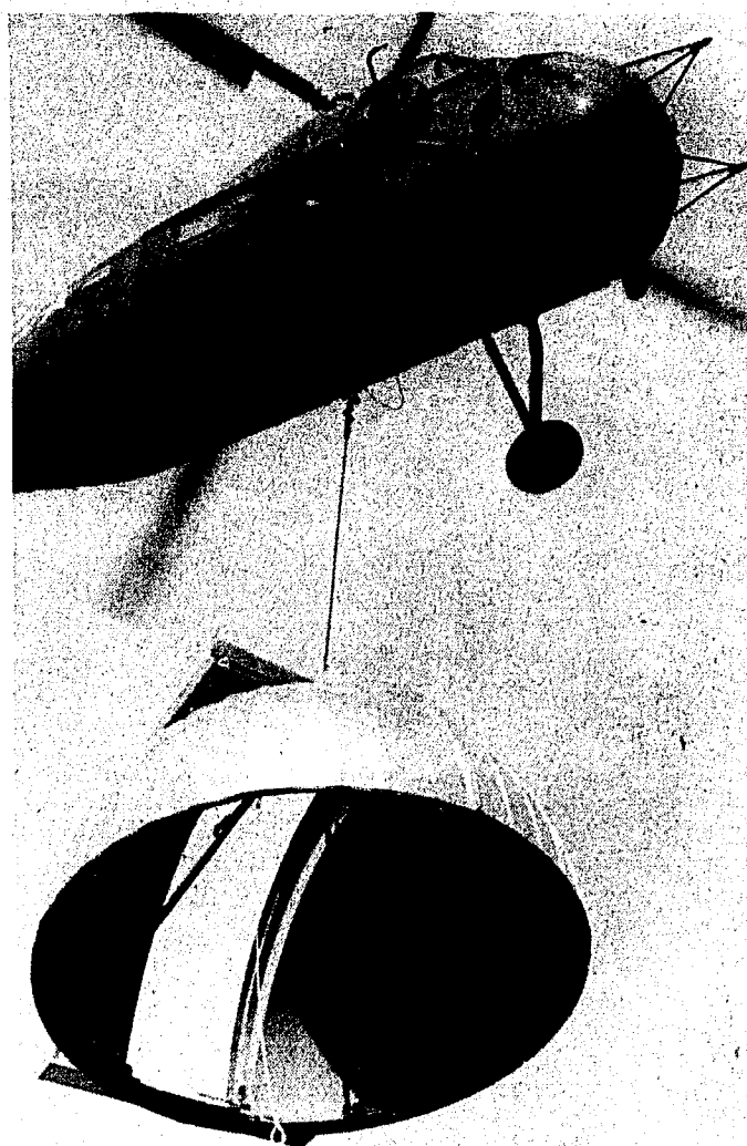
UP UP AND AWAY — The observatory dome atop the Physical Science building is moved to a new location near the golf course where the new observatory is being constructed. The helicopter used in the operation was loaned to the university for the project by the Idaho National Guard.
