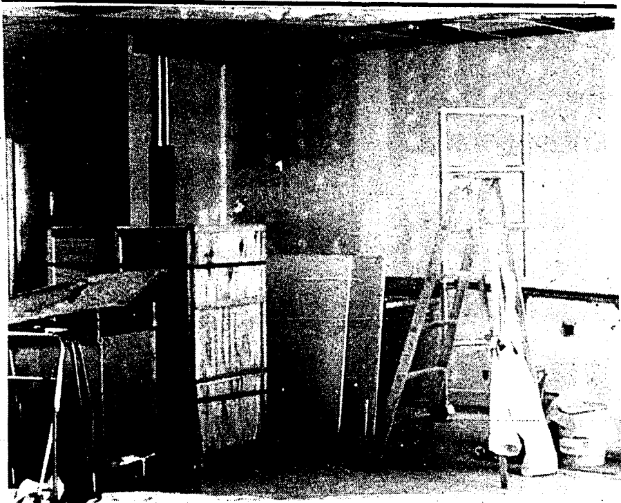
REMODELING —The small cafeteria on the east side of the Wallace Complex is being remodeled into a Snack Bar this fall. When the construction is complete, students will be able to buy a variety of food items from 8-11:30 p.m. Monday through Thursday and 5-11:30 p.m. Sunday. These items can be bought outright or with points from meal tickets.
