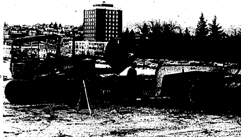
UNDER CONSTRUCTION — The new Law building, to be located West of the Physical Science Building, is now under construction.
