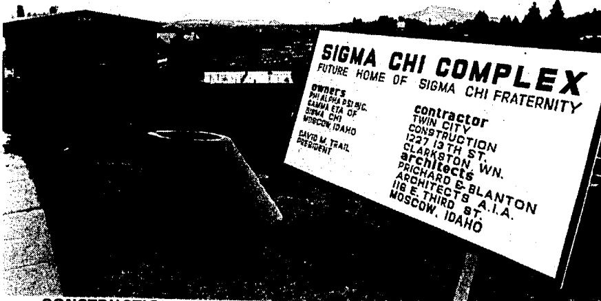
CONSTRUCTION AT THE SIGMA CHI site is progressing to meet the second semester deadline for the fraternity.
