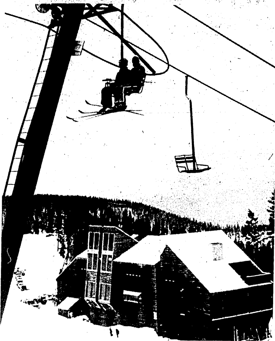
Silverhorn is served by a mile-long double chairlift which carries 750 skiers per hour up the mountain. The complete day lodge serves skiers and non-skiers alike with a cafeteria, cocktail lounge, ski shop and brown bag lounge.
