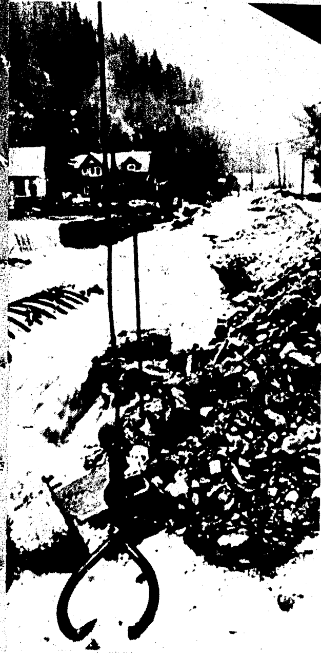
The devastating destruction of the recent floods in northern Idaho is shown in these Associated Press photos. (Above) Overflow from Placer Creek in Wallace completely ripped up this street, exposing culverts that used to be buried. (Low right) Rampaging Pine Creek opposite Pinehurst (four miles west of Kellogg) ripped chunks from the eastbound lane of
