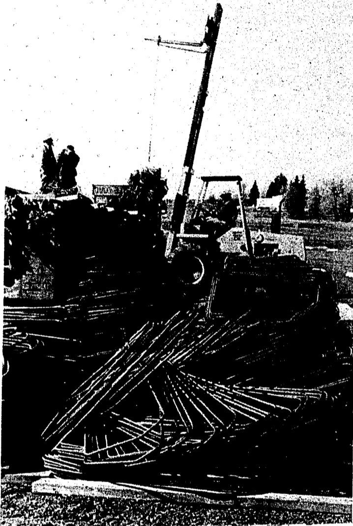
Steel beams and other structural material for the roof of the stadium arrived on campus this week and were unloaded by workmen at the stadium site Thursday afternoon. The steel is arriving by rail and being trucked through campus from the railroad tracks to the stadium.
