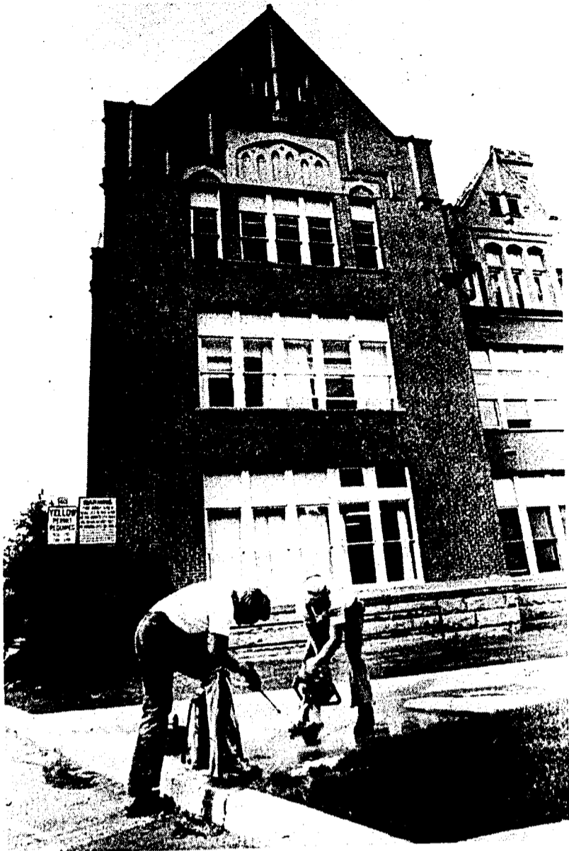
Work began yesterday by the Administration Building on curb cuts to accomodate handicapped students. The contract with Ray L. Eisinger Construction, for curb cuts, should be completed in February 1979. Photo by Mark Johann.
