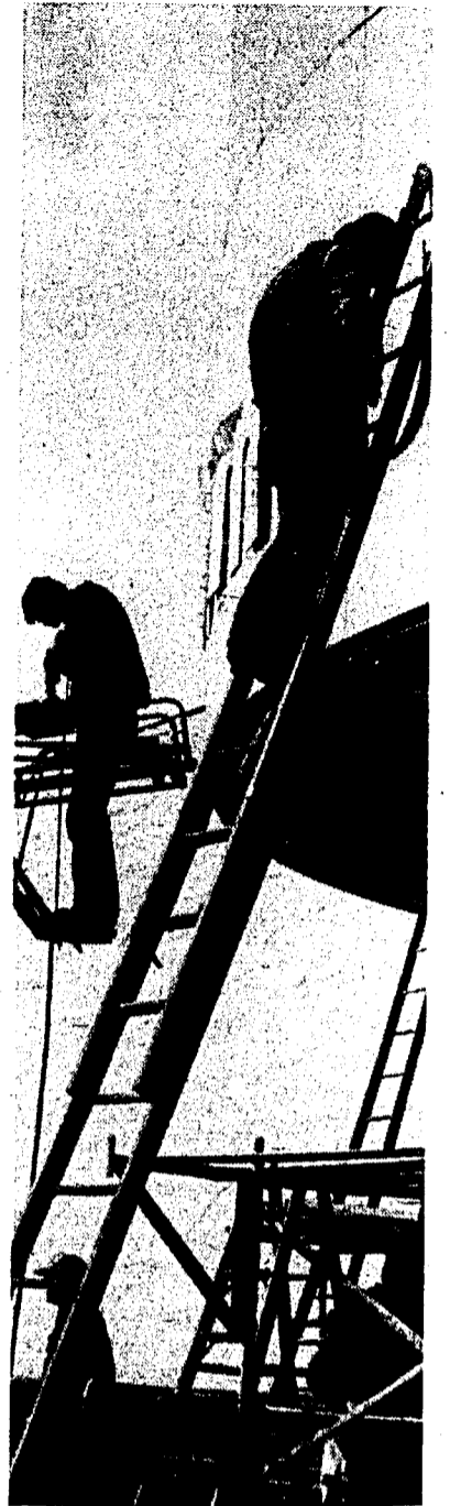
Workmen add finishing touches to the Moscow Mall. Some of the stores will open Wednesday. Photo by Jim Borden.
