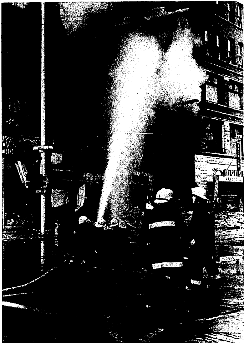
Fireman battle a blaze that gutted Spokane's historic Zukor Building Sunday. One firefighter was killed and one injured when the north wall of the building collapsed. Officials suspect arson was the cause of the fire. Photo by Patrick House.
