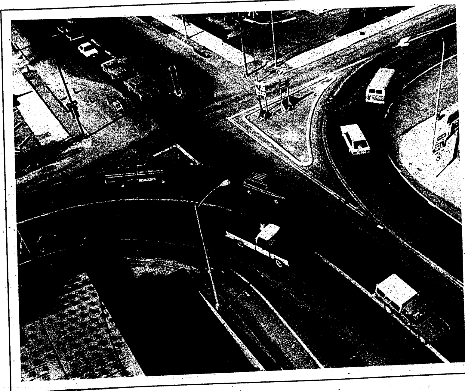
Workers braved hot summer sun to revitalize downtown Moscow and reroute traffic.
