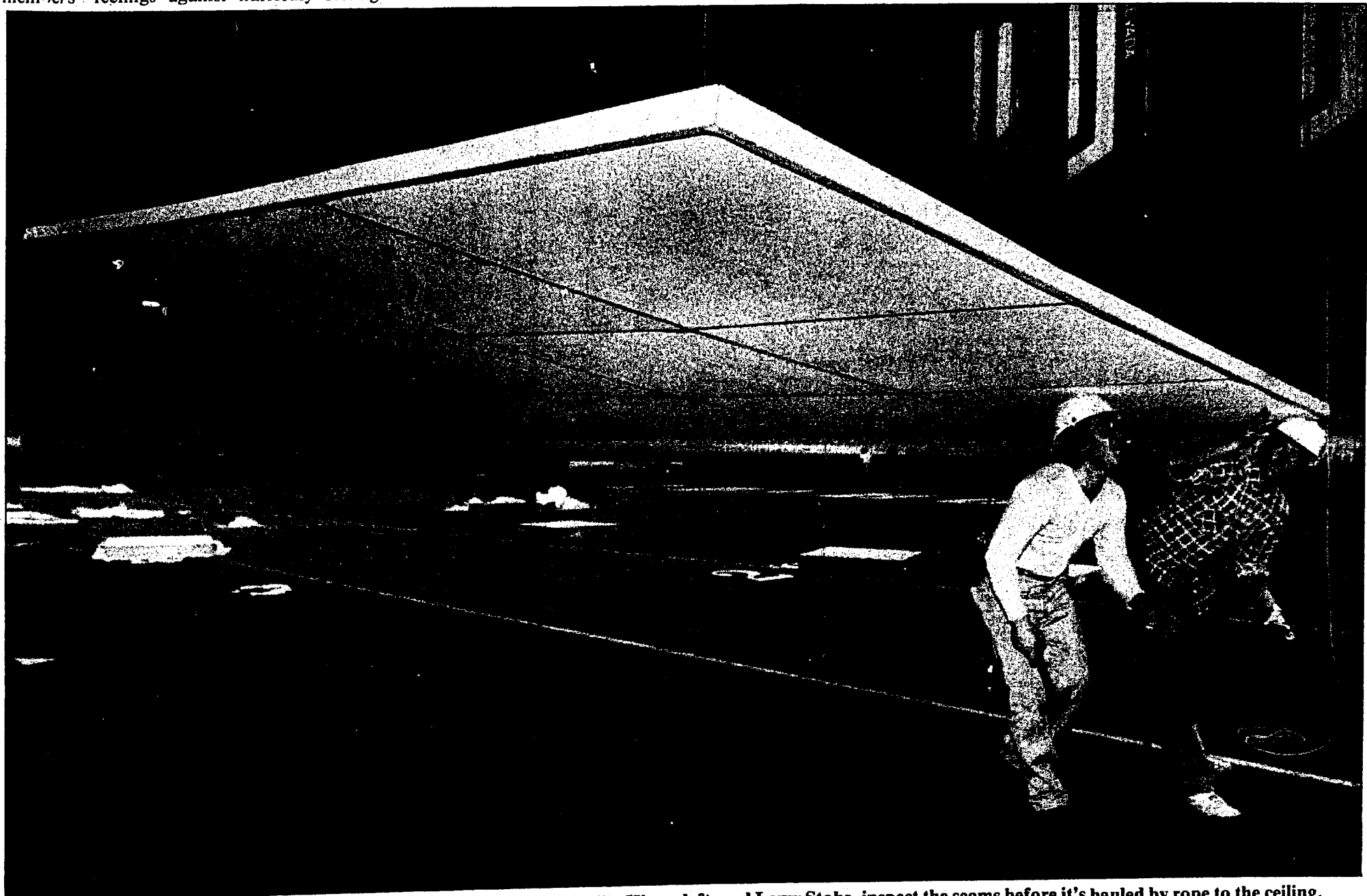
Acoustic tiles go up as if by magic during work in the dome Thursday. Mike Hines, left, and Larry Stohs, inspect the seams before it's hauled by rope to the ceiling.
