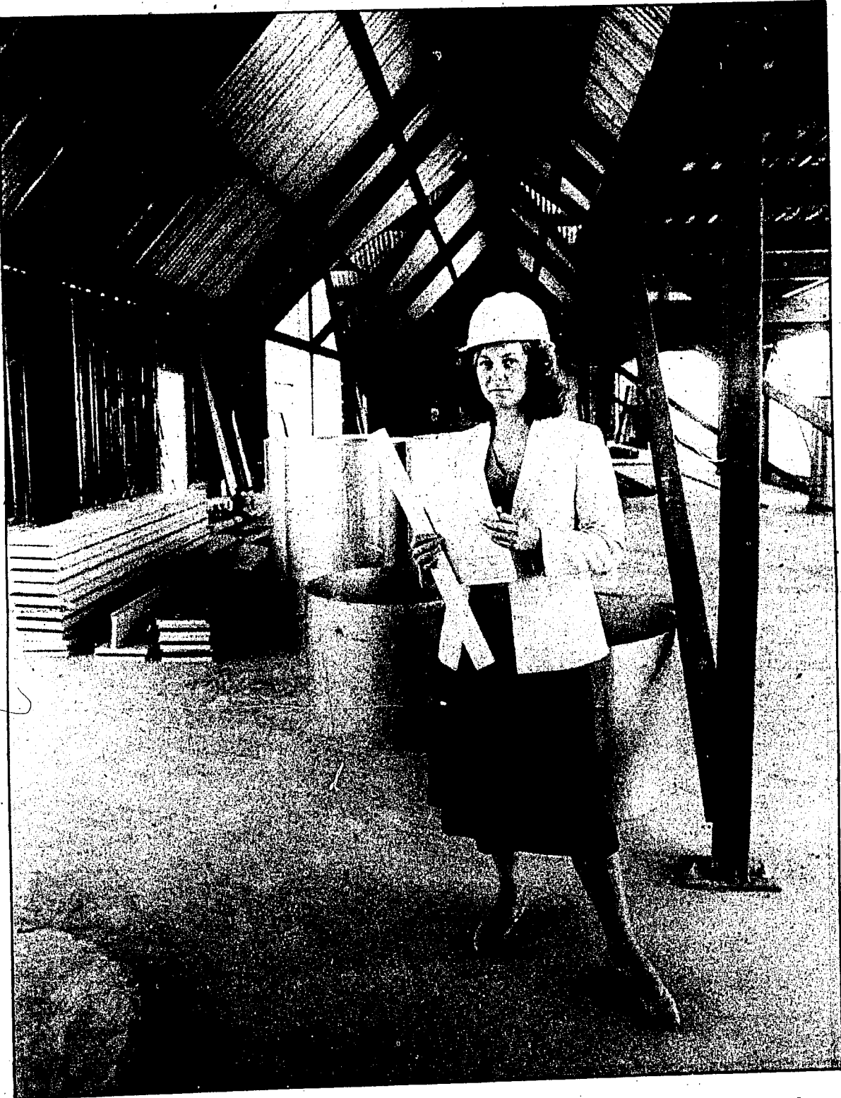
The new Director of Facility Planning, Joanne Reece monitors the progress of construction at the new Life Science Building. Photo Bureau/Deb Gilbertson
