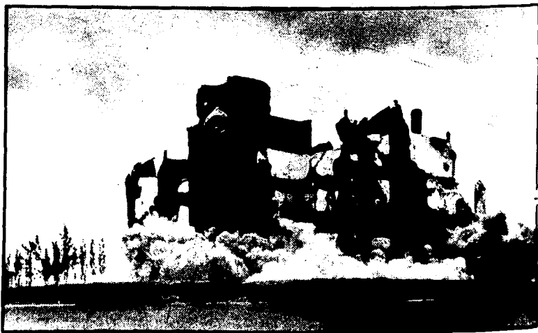
DYNAMITE crumbled the walls of the 1906 Administration Building after a fire gutted the building. (No. 1-51-30a Photo Collection, University of Idaho Library)
