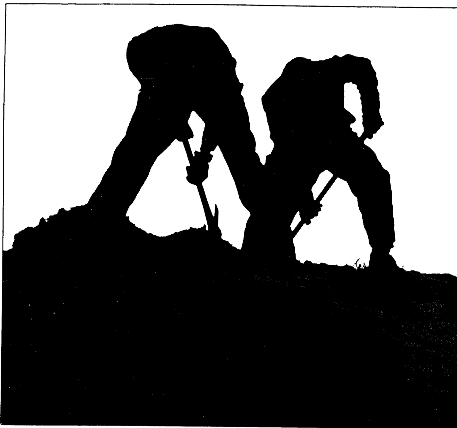
Doug Hayes (left) and Jerry Hamilton get in some last minute digging before the sun drops below the horizon. They are digging a hole for a new light post to be put at the top of the stairs leading to the Kibbie Dome.
