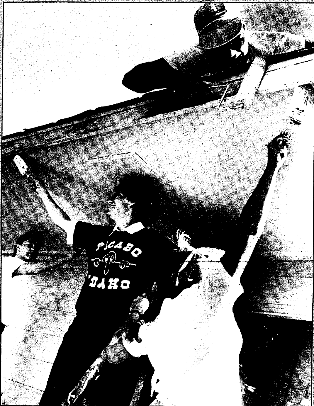
PITCHING IN TO PAINT. Allison Lindholm (far left), President Zinser, Martha Schell and Bruce Lowther (on roof) work together to finish painting a house Saturday afternoon. (BRIAN JOHNSON PHOTO)
